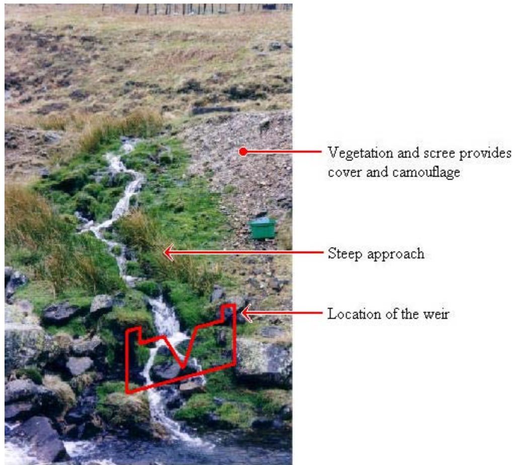
Figure 3.4 a photograph showing the Mine Adit and where the weir will be located, the concrete flanks of the weir will be set into the bank and therefore remain hidden by the scree and vegetation.
