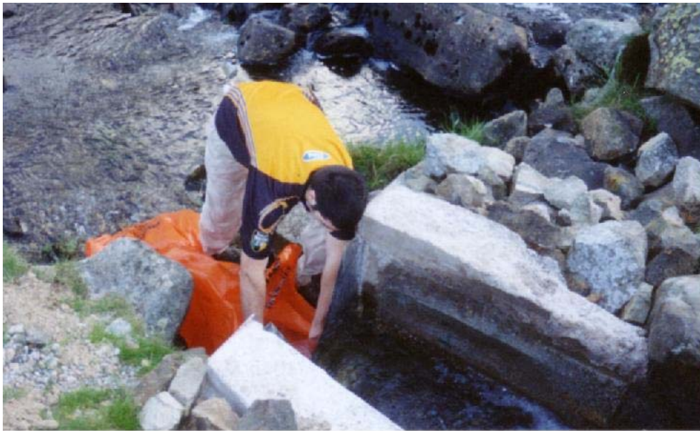
Figure 4.1, a photo showing volumetric gauging being carried out at the weir in the Mine Adit.
