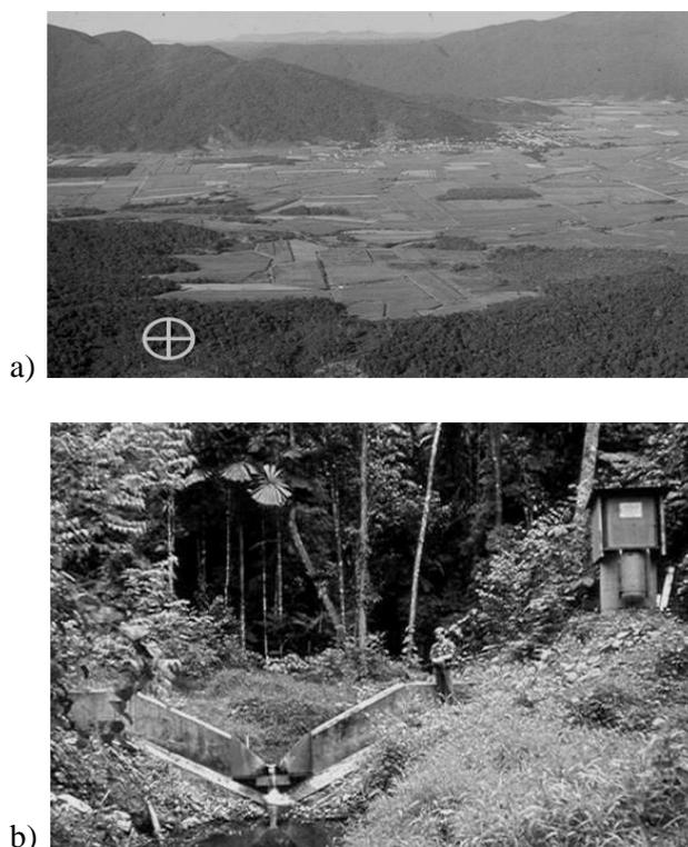
**Fig. 1** The South Creek Experimental Catchment at  $17^{\circ} 20' S$   $145^{\circ} 59' E$ , a) shown with a white cross in the foreground and located near to Babinda town visible in the background, and b) gauged with a compound V-notch weir.
