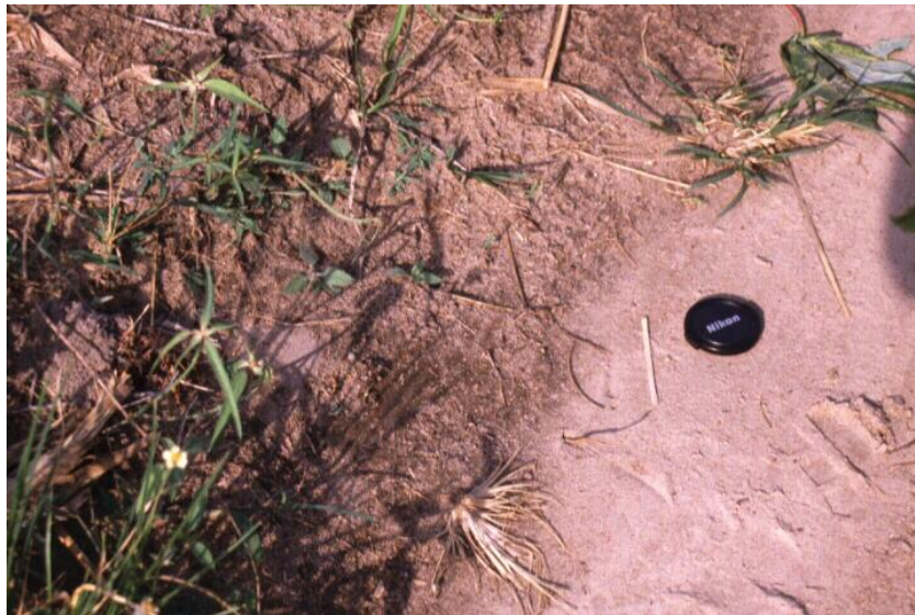
Figure 8. Loose sand surface of path 1, Adabra village
