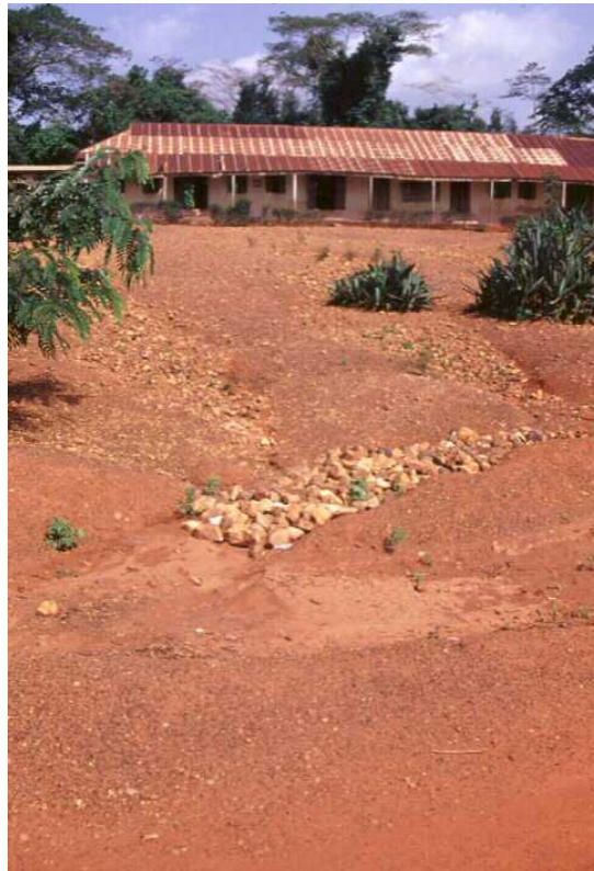
Figure 17. Gully control using rock dams, school grounds, Sampa village
