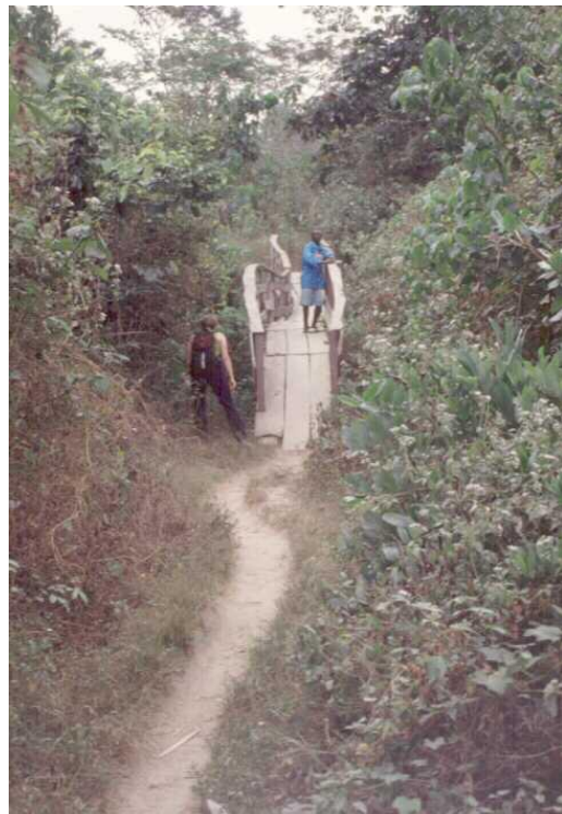
Figure 27. The cedar bridge constructed by the community along Path 2, Awurabo village
