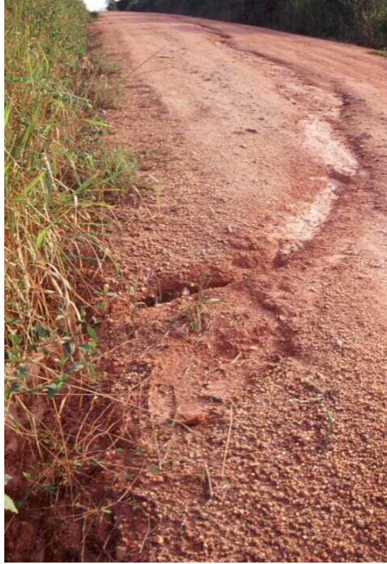
Figure 6. Road gully developed on the slope on the far slope in Figure 5, Adabra village
