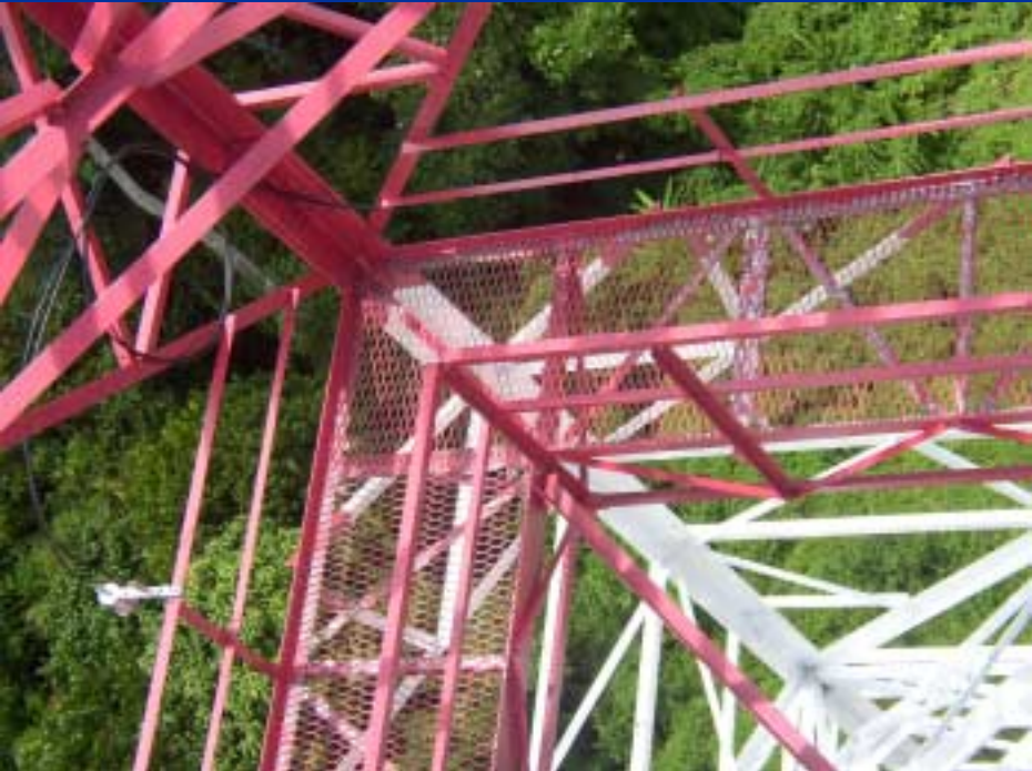
A 100 metre instrumented tower with air intakes at 30, 60 & 100 m
